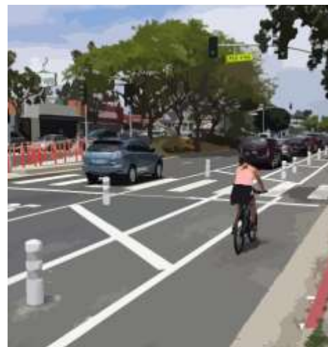
Fig. 7 Traffic control devices and pedestrian safety caution signs
