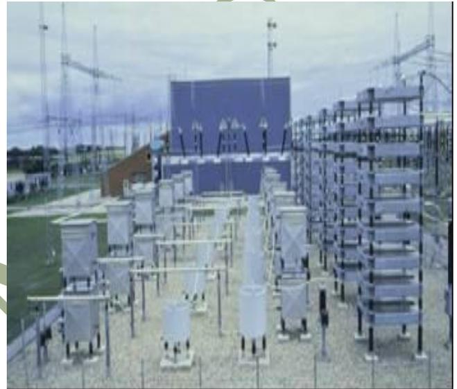
Fig. 1. HVDC converter station with AC filters in the foreground and valve hall in the background
