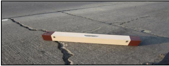
Fig Pavement distress on Expressway
