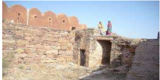
PHOTO-2 Conservation Work on Fort Wall
