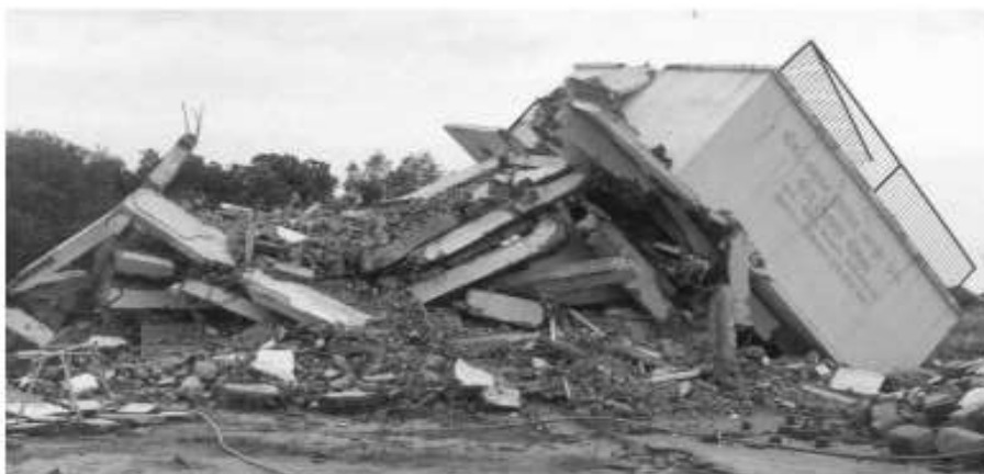
Fig.3 Staging Collapse in Manfera village
