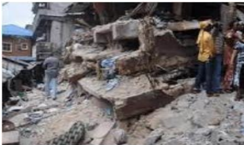
Figure 2.2: 10 killed, 23 rescued in Lagos three-storey building collapse
