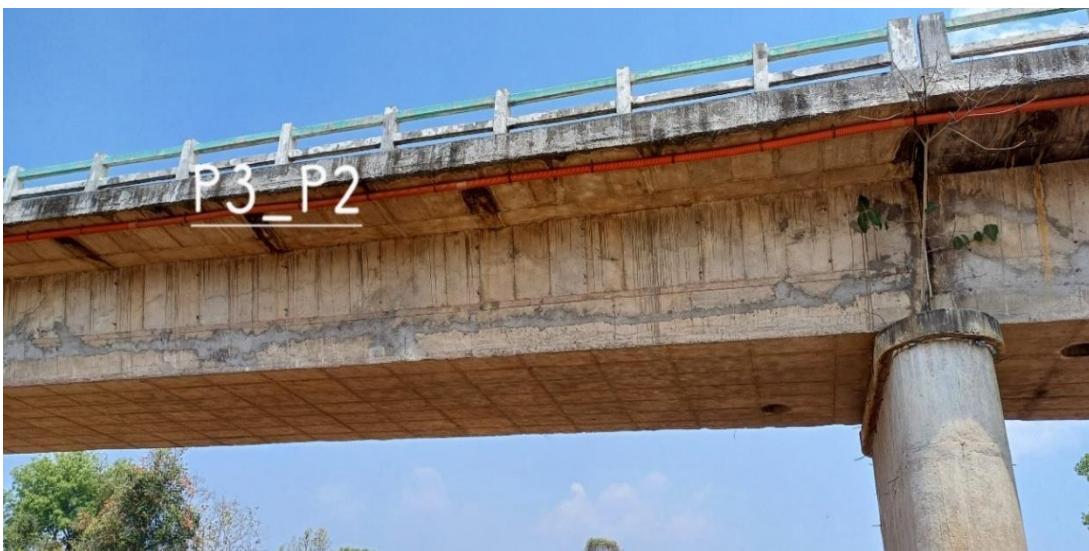
Fig.2. Site condition connecting pier-P2 to pier-P3
