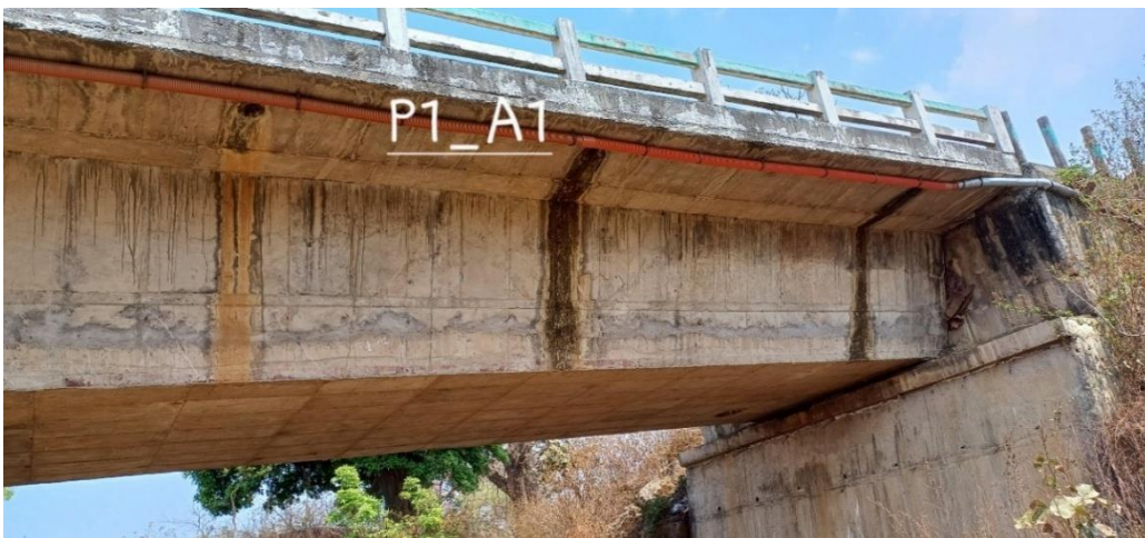
Fig.1. Site condition connecting abutment-A1 to pier-P1
