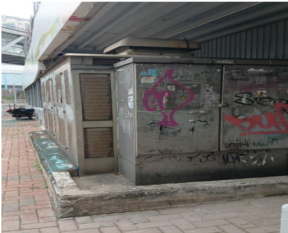
Figure 2: Concrete plinth provided with 4 inches high kerb
