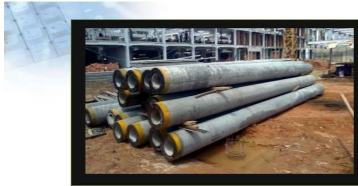
Figure 1. Spun Pile diameter 30 cm, length 6 meters,
