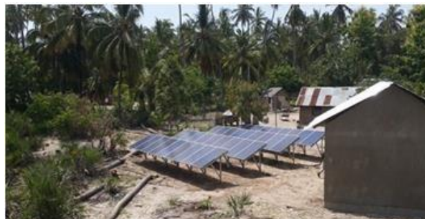
Figure 1(c): OPZs battery bank, Inverter and charge controllers in the Power House in Kuruti Island
