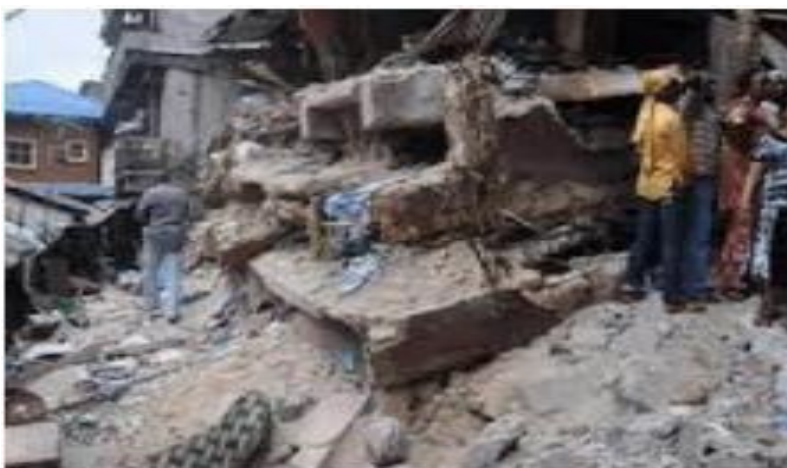
Figure 2.2: 10 killed, 23 rescued in Lagos three-storey building collapse
