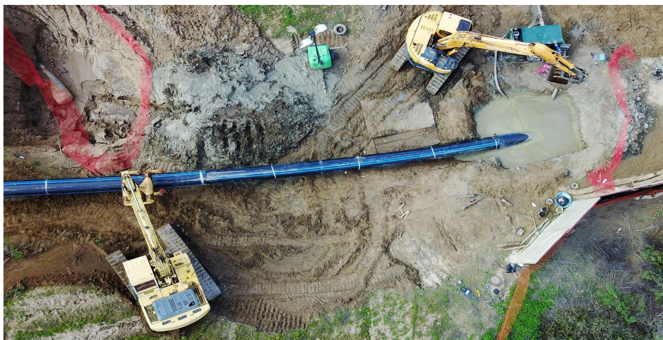
Fig 7. Arial view of HDD Process [21]
