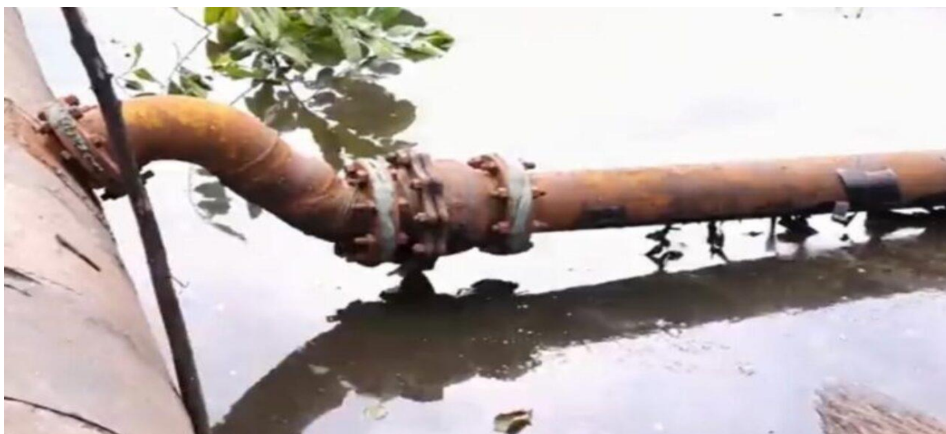
Fig 1 showing a tap of point on a crude line made by vandals [8]
