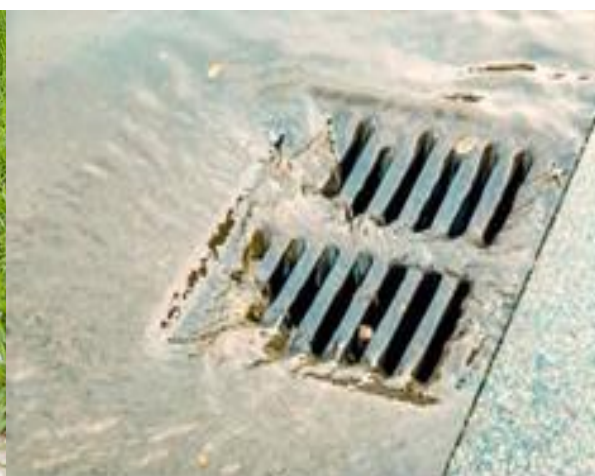
Enclosed Manhole at Utako
