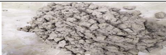
Figure 2.18: Cement, sand, stone and water mixing
