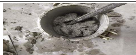
Figure 2.19: Compacting the mixture
