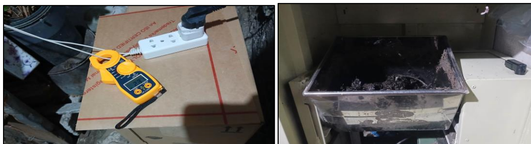
Figure 3 Setup During the Ampere Rating Test
