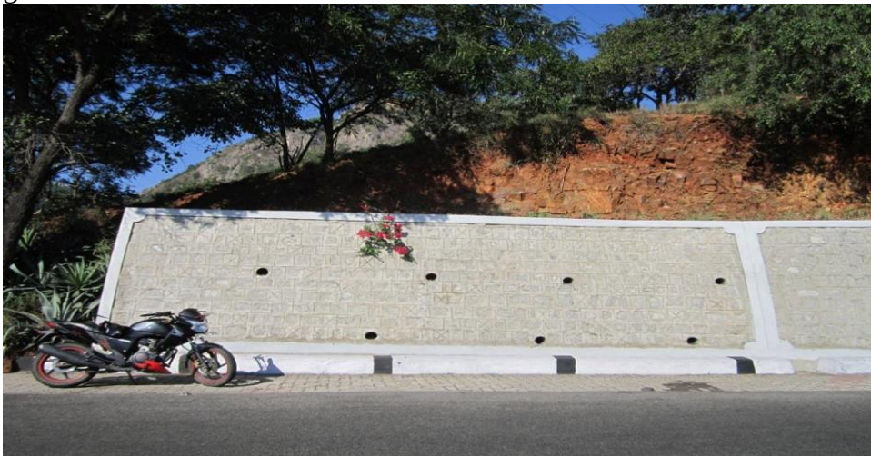
Fig. 11: A rock-wall protection wall was constructed along the Tirupati-Tirumala second ghat road using Peruru granite
