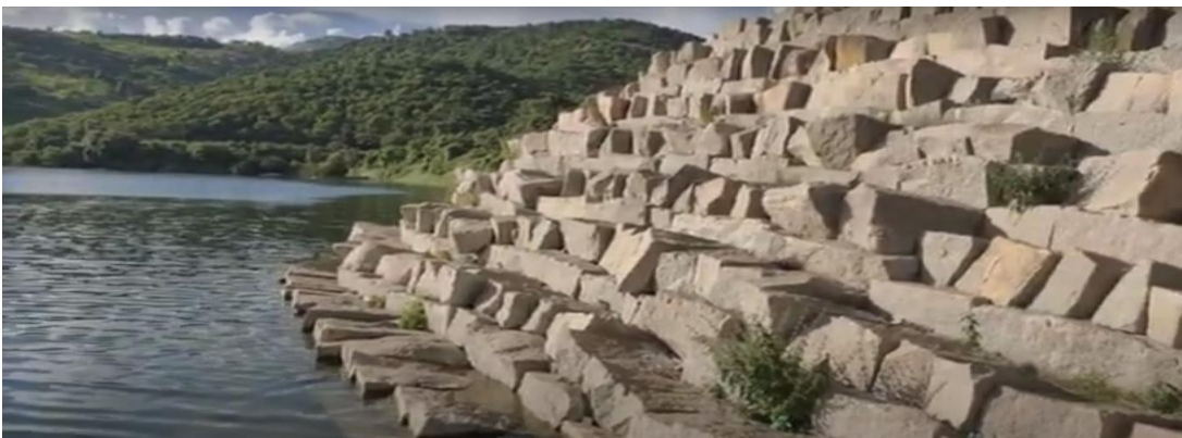
Fig. 8: The compound wall of Govindarajaswamy temple at Tirupati was constructed using Peruru granite
