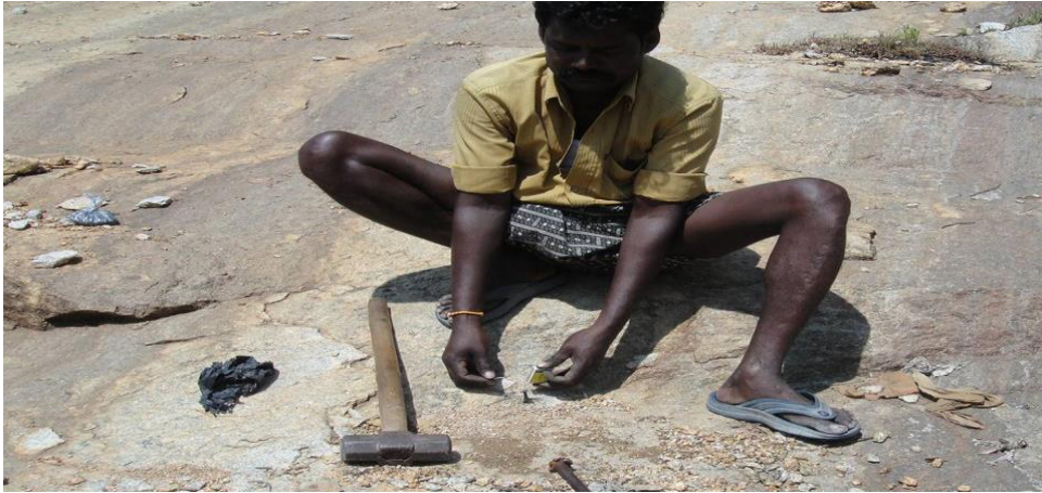
Fig. 4: Making road metal using a hammer
