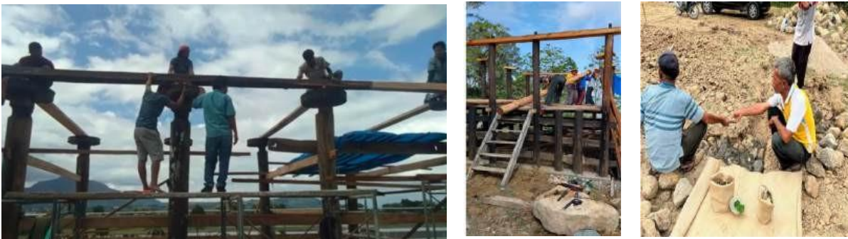
Figure 6. The lower structure and pillars of a house on stilts
