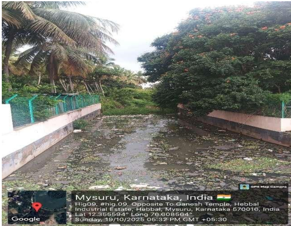
Figure 4: Storm Water Drains, Mysore
