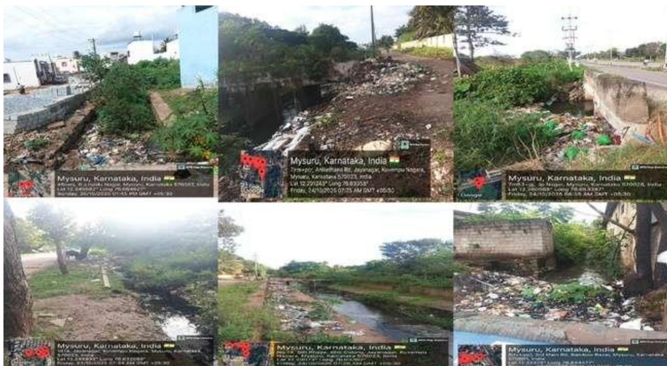
Figure 2: Storm Water Drains, Mysore
