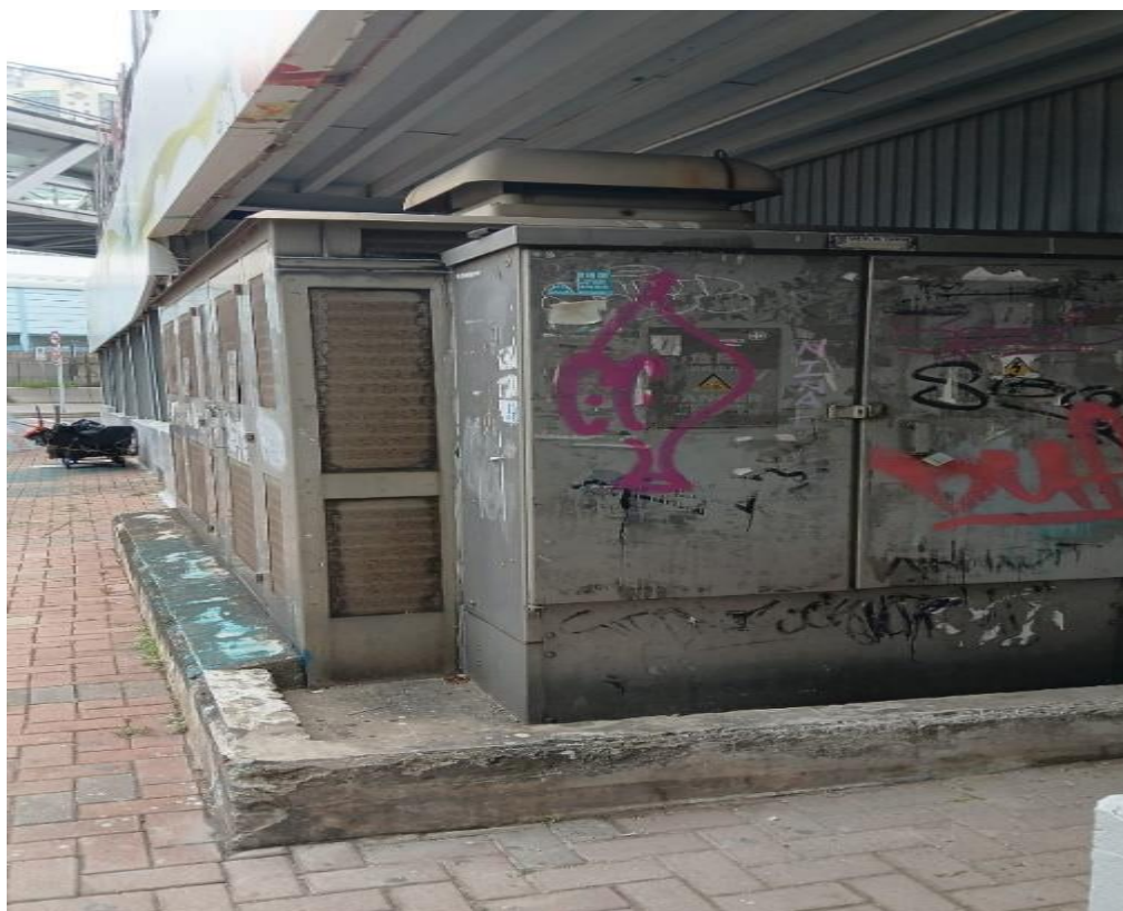
Figure 2: Concrete plinth provided with 4 inches high kerb
